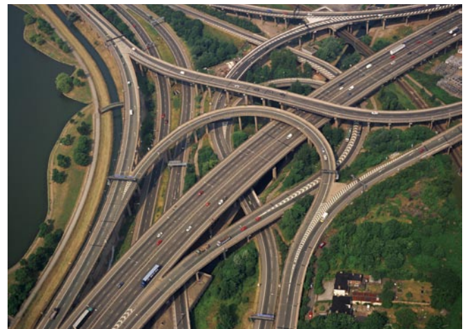
The notorious Spaghetti junction on M6 is part of the motorway system encircling Birmingham.
